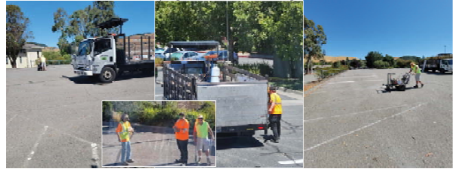
Striping of St. Isabella Parking Lot
